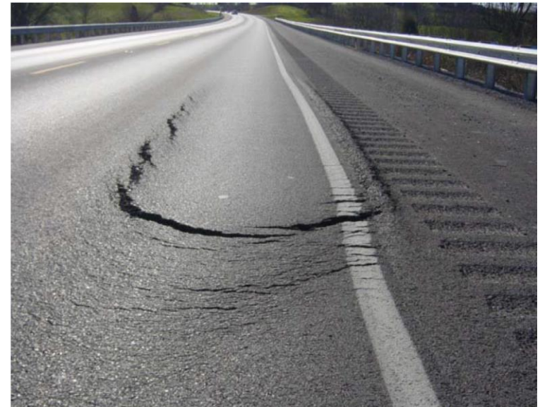
Slippage cracking
