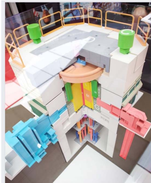
Idaho National Laboratory's Transient Reactor Test Facility, commonly referred to as TREAT, is an air-cooled, thermal spectrum test facility designed to evaluate reactor fuels and structural materials. This 3D-printed model of the reactor shows a cutaway of its inner workings. | Energy Department photo by Matt Dozier.
